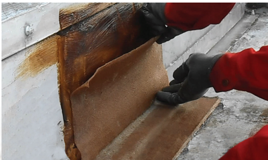
Advantageous in providing long-lasting protection to the corrosion vulnerable areas of tank chimes.
